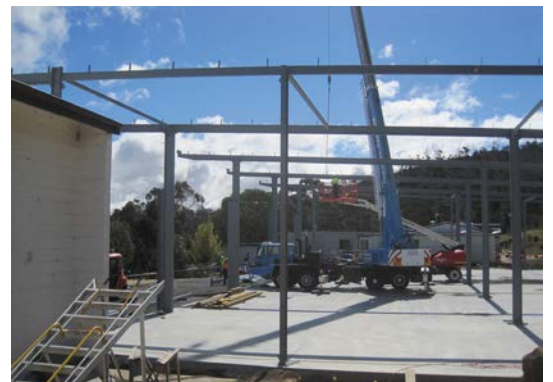
Construction in progress.
